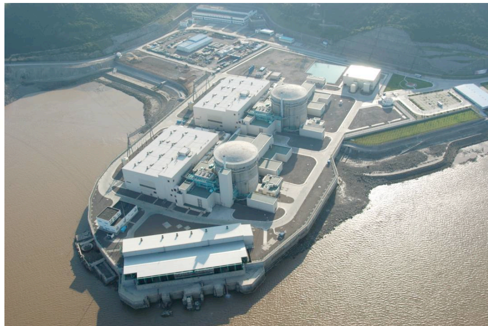
Qinshan Phase III site – Twin CANDU 6 Units
