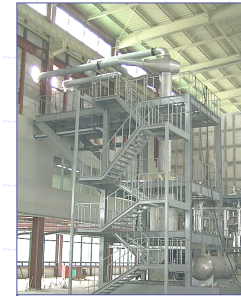
PVCS Experimental Facility
