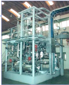
Thermal Hydraulic Experimental Facility
