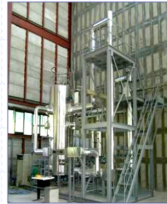
Water Mock-up Experimental Facility
